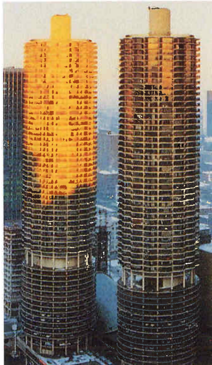
A set of Voss Bearing pads will support each of these twin T's in the construction of this new parking garage in Chicagoland.
